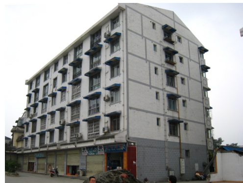
Fig. (2). Typical confined masonry buildings in Sichuan.
