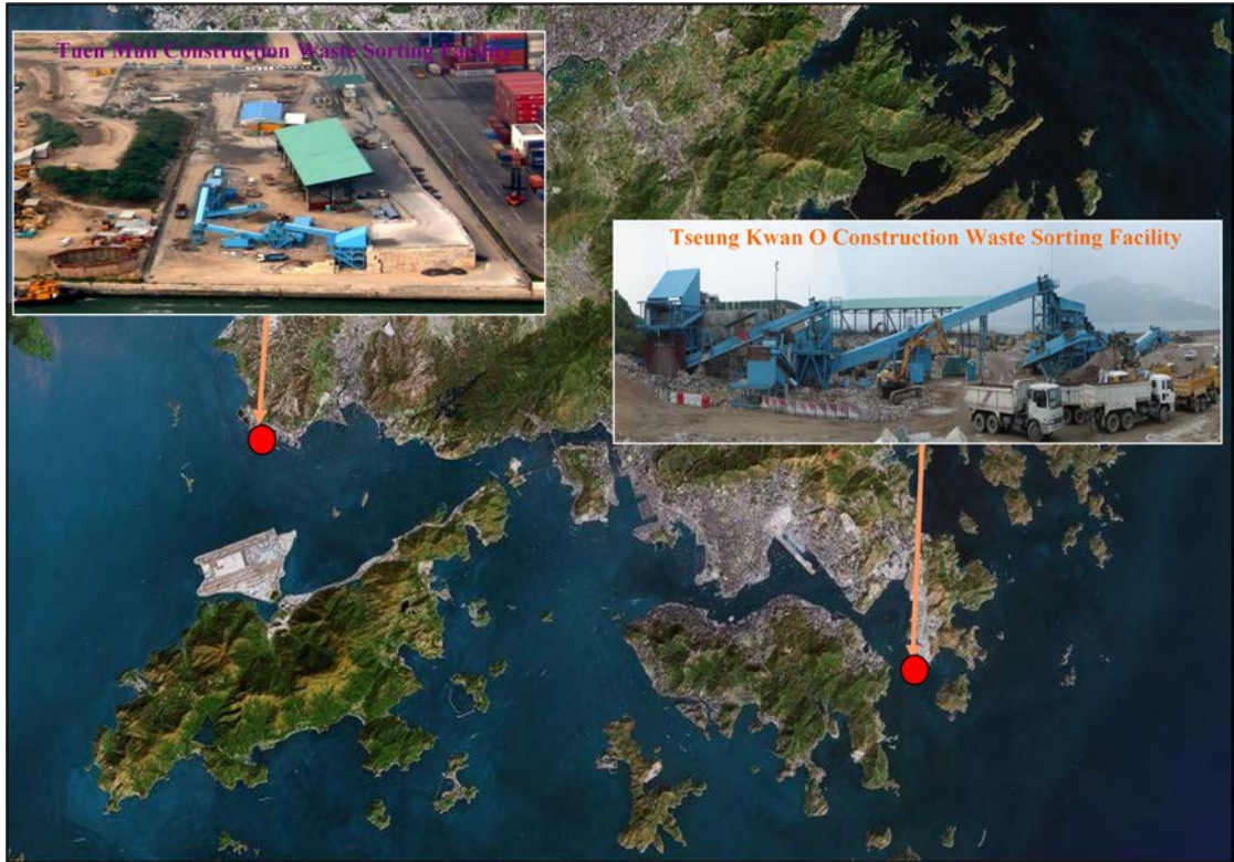
Figure 3: Two construction waste sorting facilities in Hong Kong [34]
