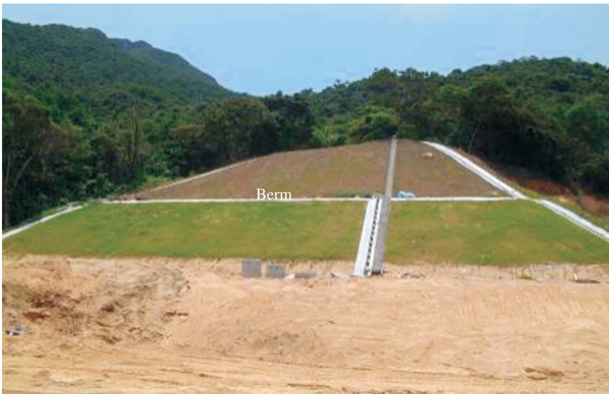
Fig. 4. Site photograph showing the cut slope and hillside slope condition after road excavation in December 2001.
