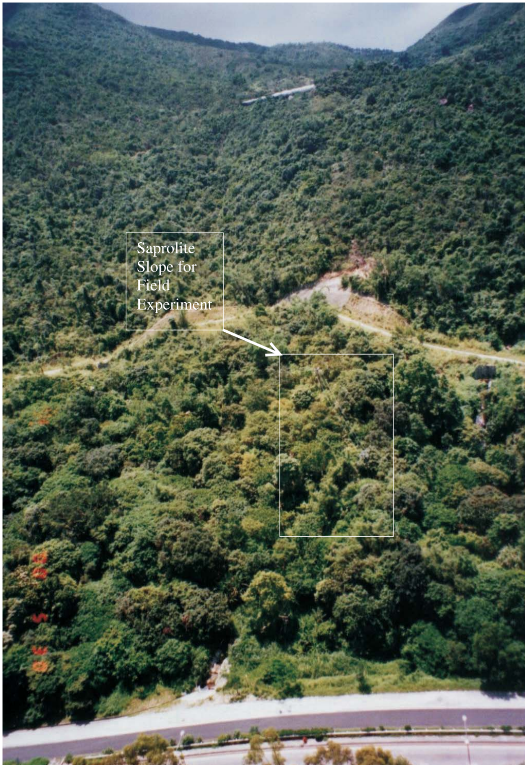
Fig. 1. Site photograph showing the hillside slope condition before road excavation in 2000.
