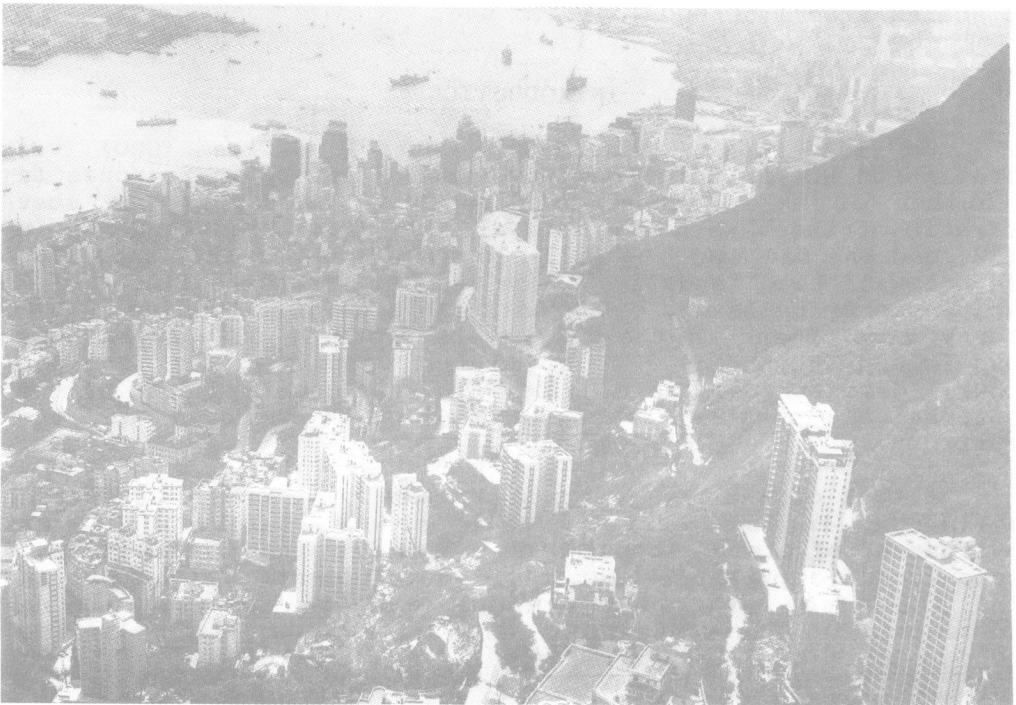
Figure 1 - An oblique aerial photograph looking east across the Mid-levels district of Hong Kong Island in June 1972. The area is intensively developed and the Kotewall Road landslip is in the foreground.
