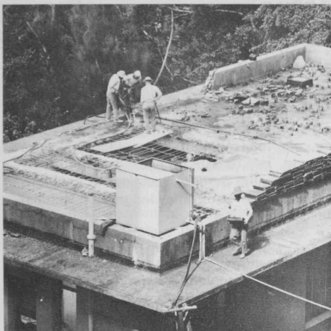
Demolition of the old Autopsy room.
