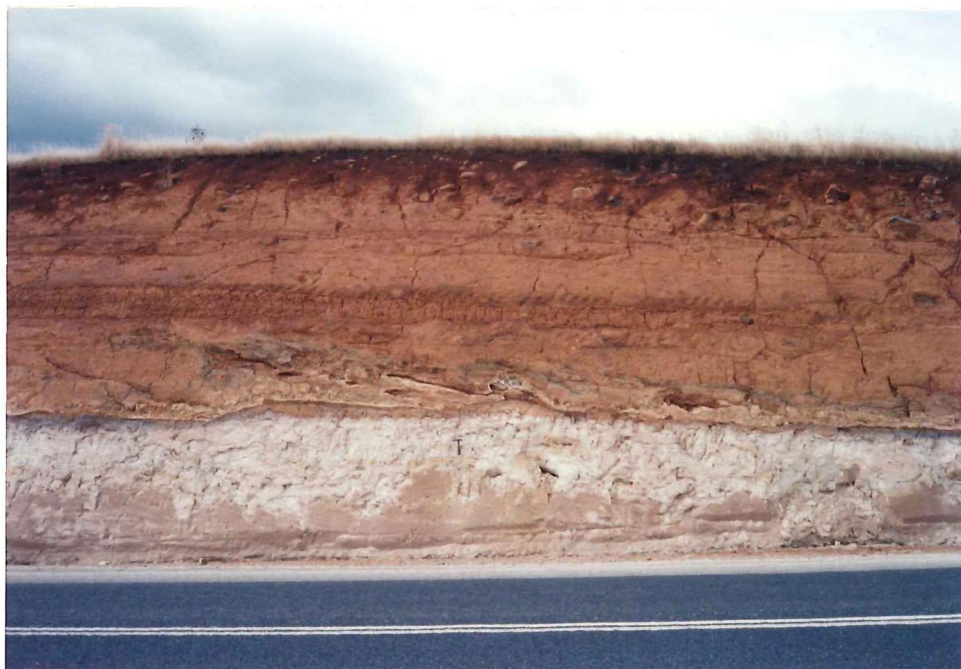
Plate 2.1 Road-cut exposure near Branhholm showing the Tertiary basalt-sediment interface. The basalt probably of Middle Miocene age is lateritized.
