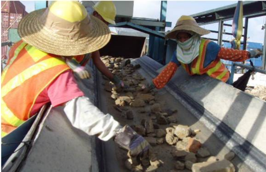
Figure 7: A snapshot of construction waste handpicking
