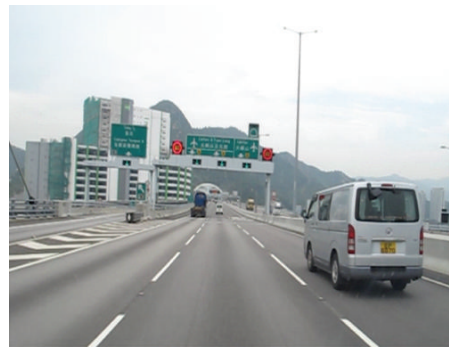
(A2) Exit of the Stonecutters Bridge is surrounded by buildings on both sides before approaching a tunnel
