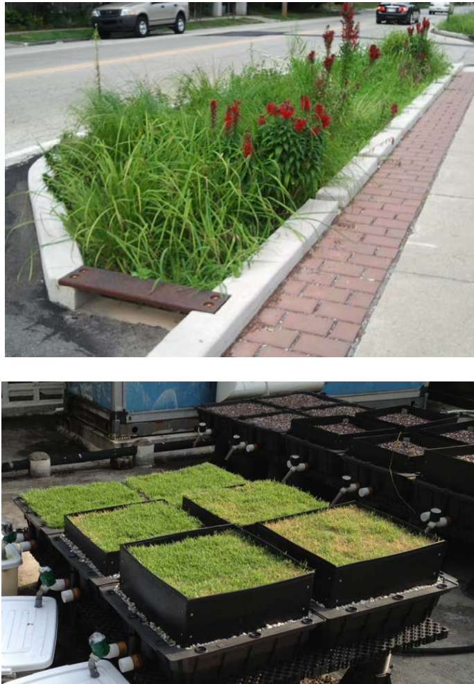
Figure 1: Examples of low impact development elements. Bioretention system (top) and green roof (bottom).
