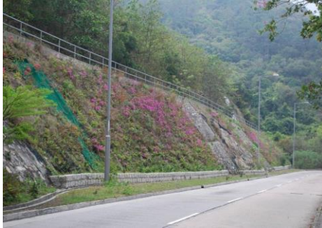
Re-planted slope, Sai Kung
