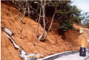
Coir erosion control matting
