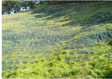
Geotextile erosion control matting
