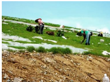
Problems of working on slopes SENT landfill restoration works
