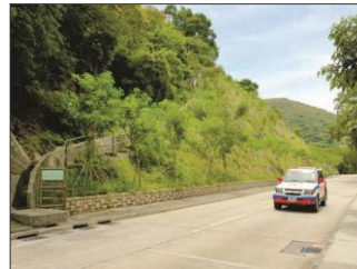
Slope planting, Sai Kung
