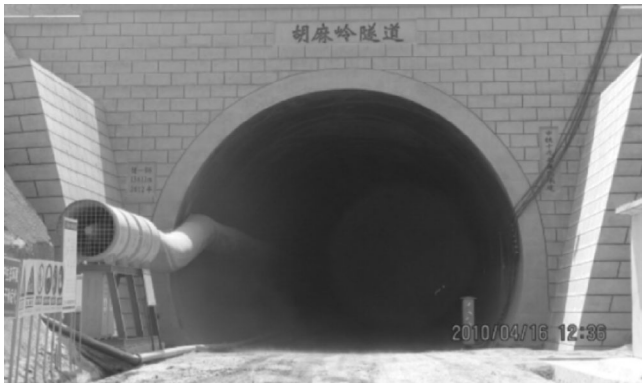
Figure 1. North portal of the Hu Maling tunnel
