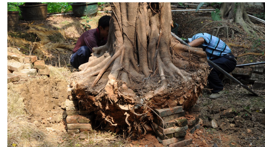
Tree set on bricks before root ball walls constructed around what is left of the roots
