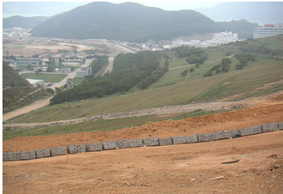
2003 - Restoration Phases 1-4. Phased planting blocks can be clearly identified as the landfill grows.
