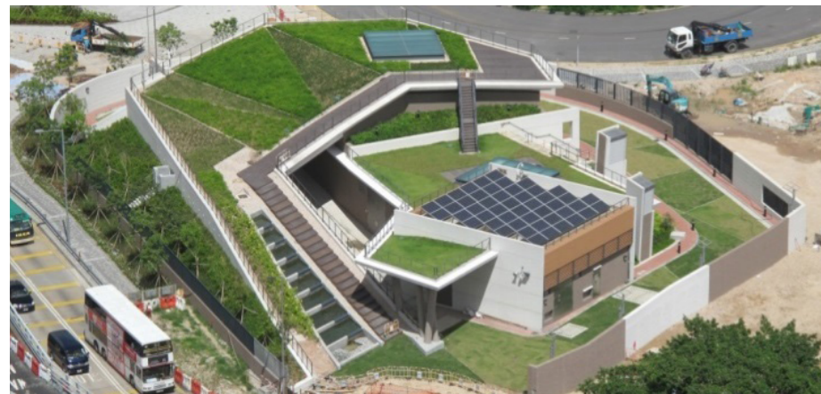
Kowloon City Pumping Station (Source: Drainage Service Department)
