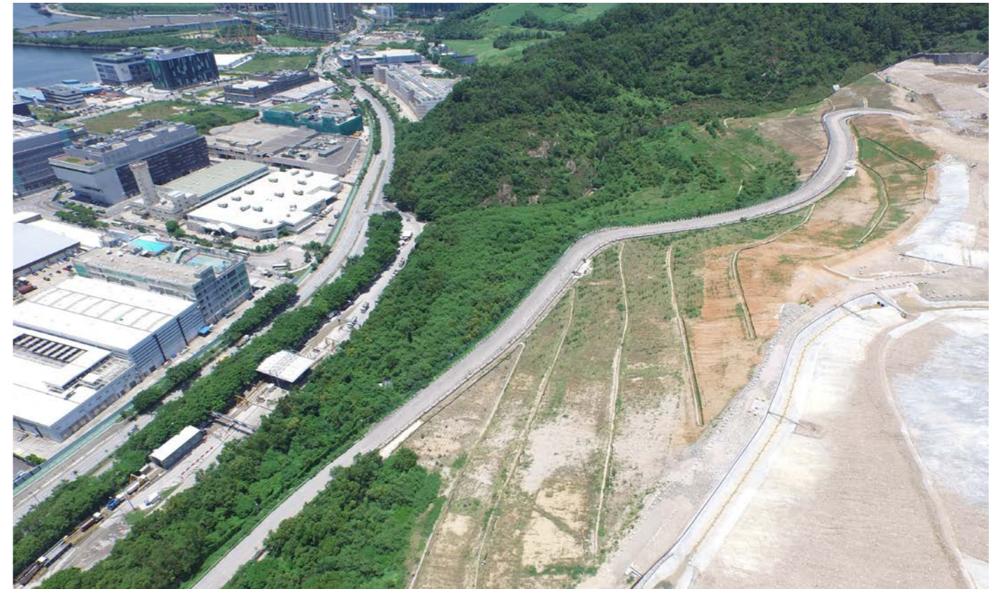
Site of SENT Landfill and adjacent Tseung Kwan O Industrial Estate
