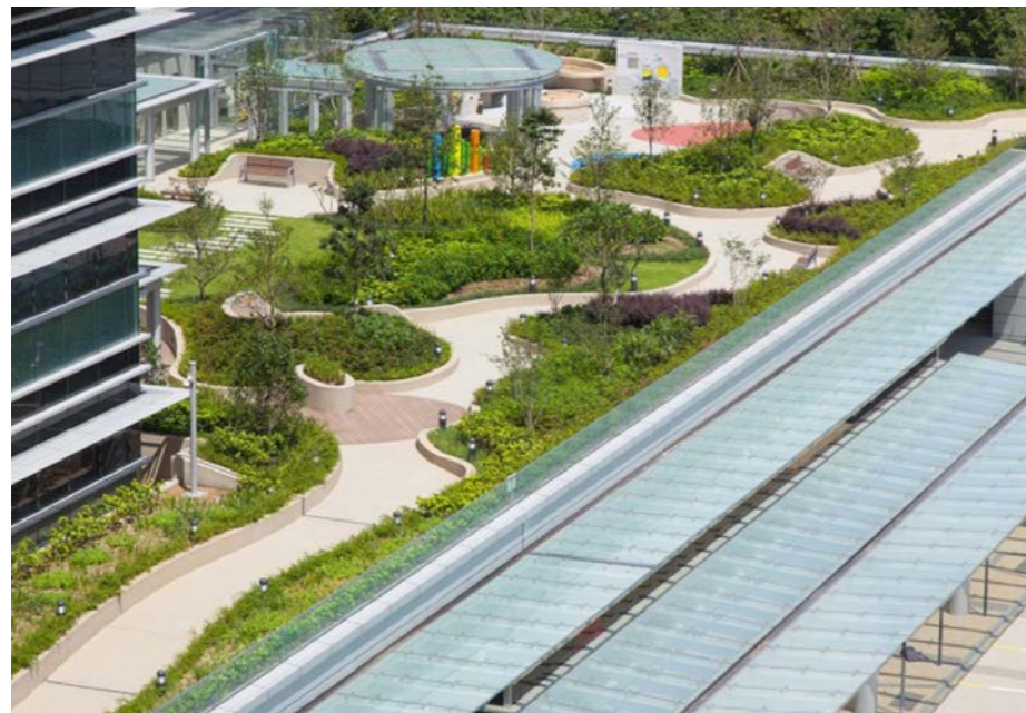
North Lantau Hospital (Source: Architectural Service Department)
