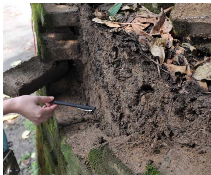
Brick wall structure containing the backfill soil
