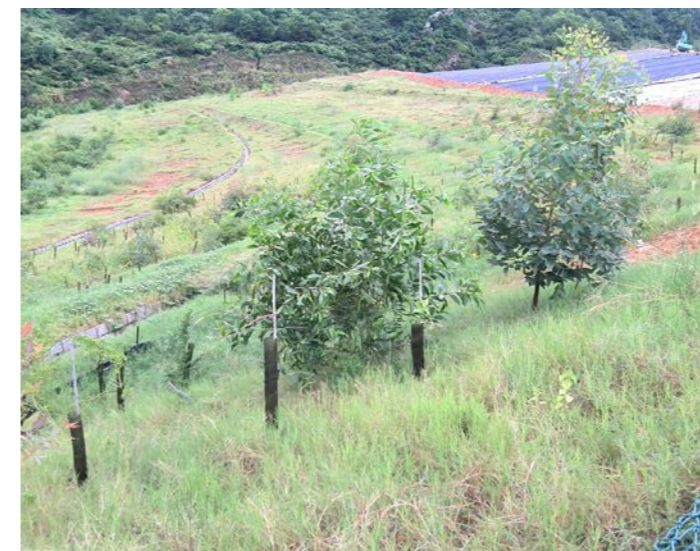
2014 - Restoration phase 9. 1500mm planting medium being graded for future planting phase
