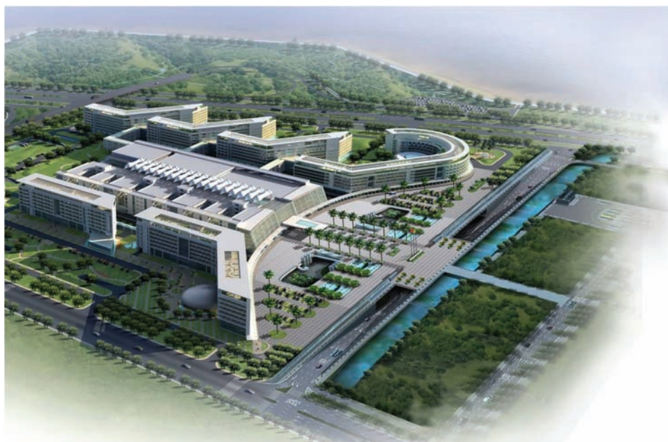
Fig 1. Hong Kong Shenzhen Hospital, 2014.
