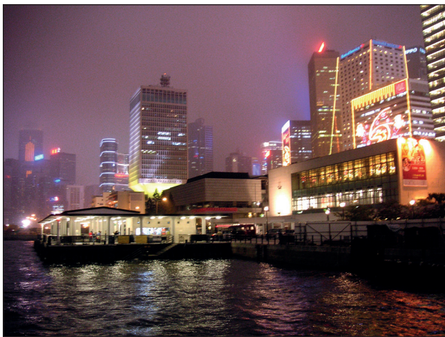
Figure 3. Queen's Pier in Hong Kong shortly before it was demolished in 2008 (CC BY-SA 2.5, see https://commons.wikimedia.org/w/index.php?curid=524247 )
