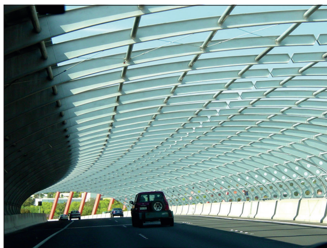
Figure 6. Flemington noise barrier on the City Link tolled motorway network in Melbourne, Australia, which opened in 1999 (by Atlantica (en wiki) (GNU Free Documentation License, see http://www.gnu.org/copyleft/fdl.html or CC-BY-SA-3.0, see http://creativecommons.org/licenses/by-sa/3.0/ ), via Wikimedia Commons)
