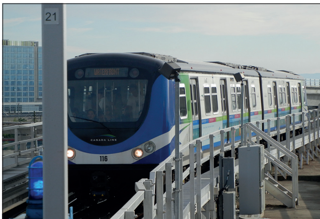
Figure 5. Bridgeport station on the Canada Line in Vancouver, Canada, which opened in 2009 (by Jeremy Andrews (own work) (CC BY-SA 3.0, see http://creativecommons.org/licenses/by-sa/3.0 ), via Wikimedia Commons)
