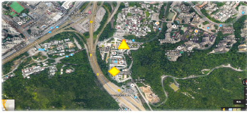
Figure 2 Two buildings in a neighborhood environment with lower building density, lower building height and larger green space
