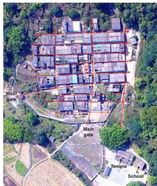
Figure 4. The layout plan of the village houses: all houses are neatly arranged along three vertical and nine horizontal lanes with the same facing direction (southeast) enclosed by the village wall according to the note given by the Feng Shui master hundred years ago to optimize living environment and control over-expansion which might exceed the carrying capacity of the landscape
