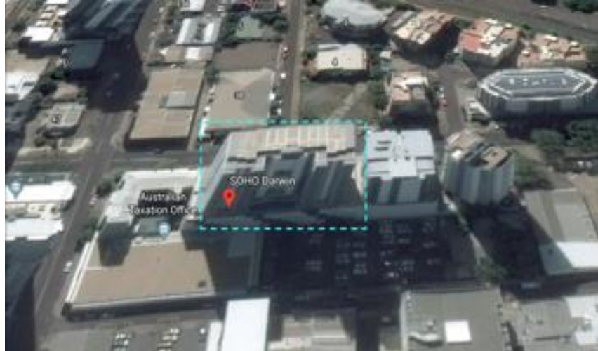
Figure 5. Existing SOHO tower from Google Earth™
