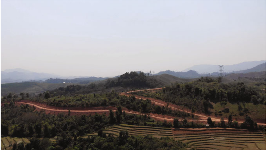
Fig. 1 Temporary access roads built for constructing remote segments and 109 tunnel portals of the China-Laos Railway. Consisting of both new construction and upgrades of existing tracks, these roads potentially increase connectivity among remote villages, but their maintenance beyond the opening date of the railway remains uncertain. Photo by Xiaoxuan Lu (March, 2019)
