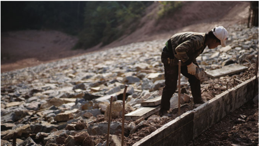
Fig. 3 A worker constructs a Vietnamese-funded irrigation dam within Nam Ha National Protected Area. Photo by Brian Cheang (March, 2019)
