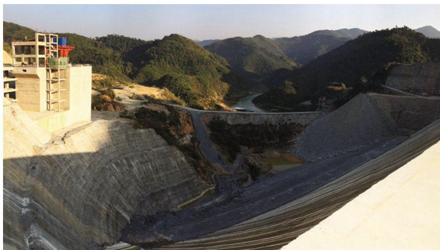
Fig. 8 Nam Tha River hydropower dam, 97% complete, which will export the majority of its generated electricity to Thailand. Photo by Ashley Scott Kelly (March, 2018)
