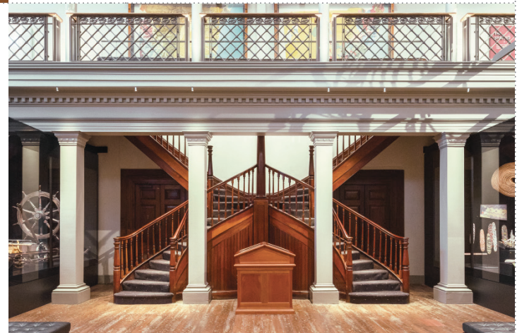
VIEW OF CONSERVED 1860s DOUBLE SPIRAL CEDAR STAIRCASE
