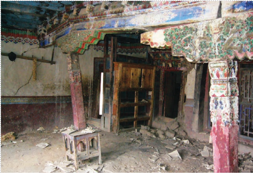
INTERIOR OF THE RABSAL ROOM SHOWING SUBSIDENCE OF PILLARS AND BEAMS
