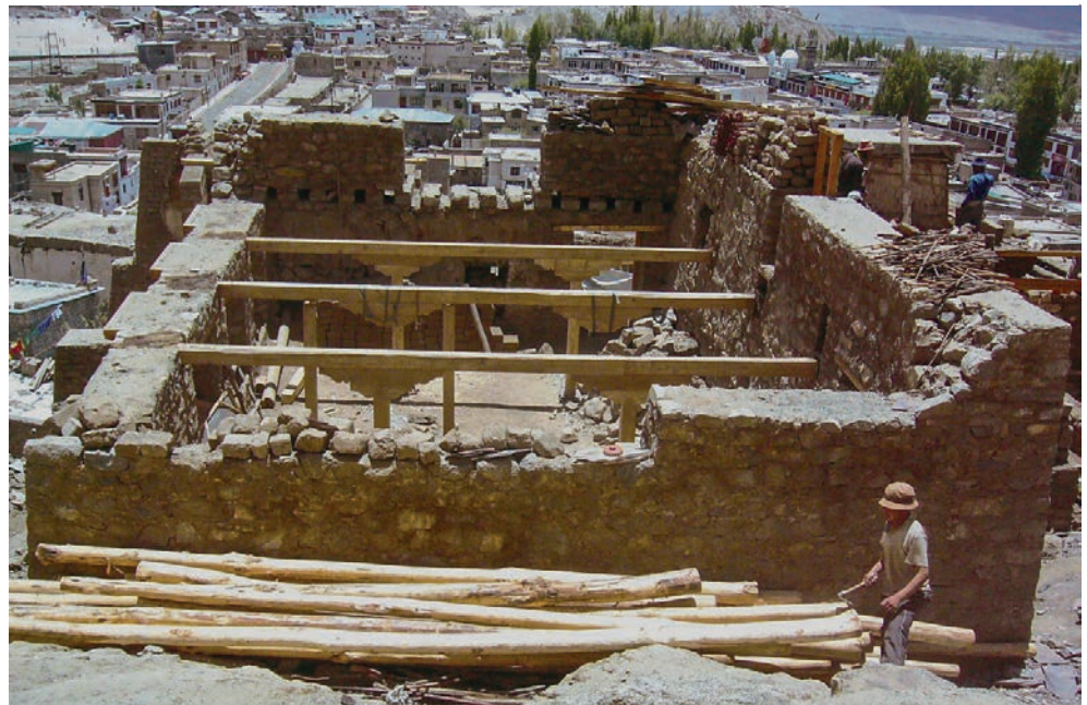
THE GROUND FLOOR WALLS WERE BUILT UP IN STONE AND THEN BRICK FOR THE UPPER FLOOR
