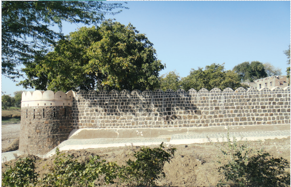
THE WALL AFTER CONSOLIDATION AND RECONSTRUCTION OF BROKEN KANGURA
