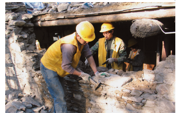
RECONSTRUCTING STONE WALL
