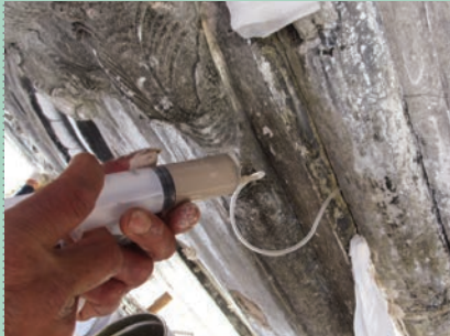
STUCCO CONSOLIDATION USING GROUT INJECTIONS
