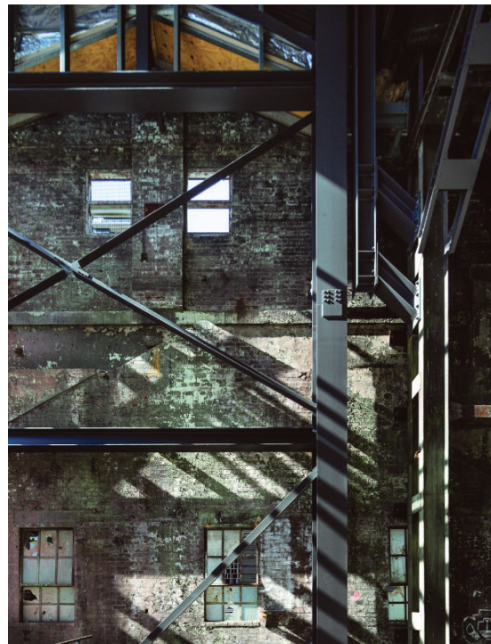
NEW STEEL SUPPORT SYSTEM
