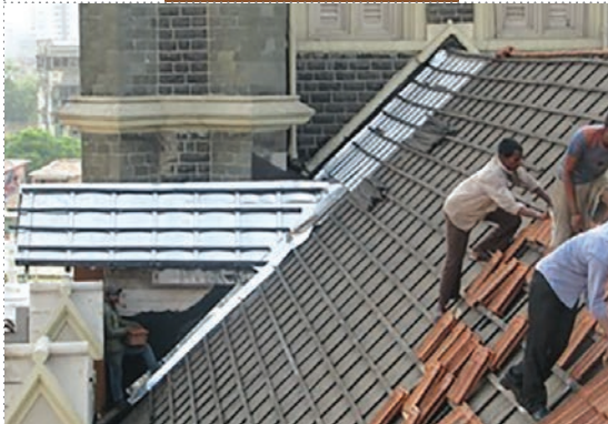
ALUMINIUM FLASHING AT ROOF JUNCTIONS
