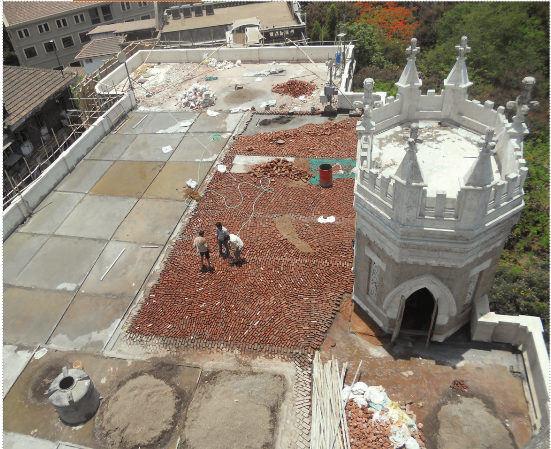
THE FLAT TERRACES WERE REDONE IN CONVENTIONAL INDIAN WATER PROOFING (BRICK BAT COBA WITH CHINA MOSAIC FINISH)
