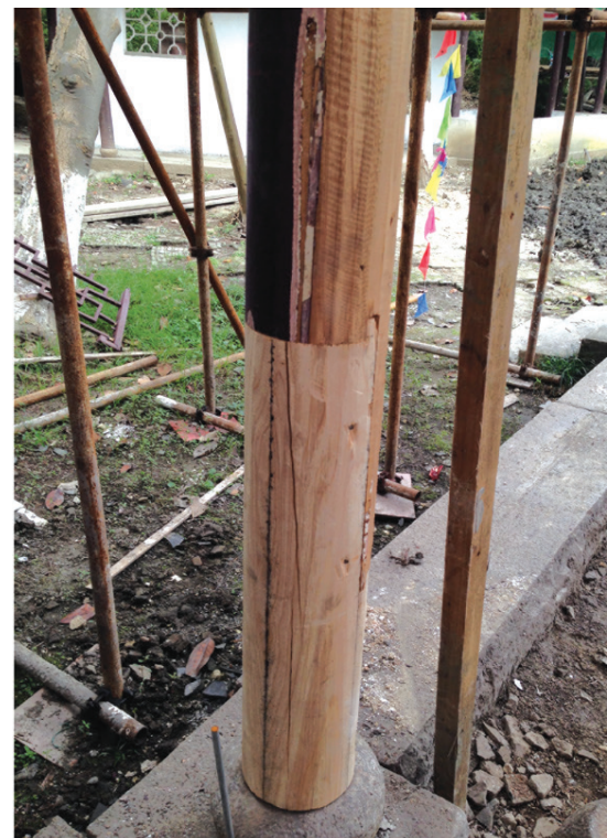
DETAILS SHOWING TECHNIQUE OF REINFORCING WOODEN PIERS
