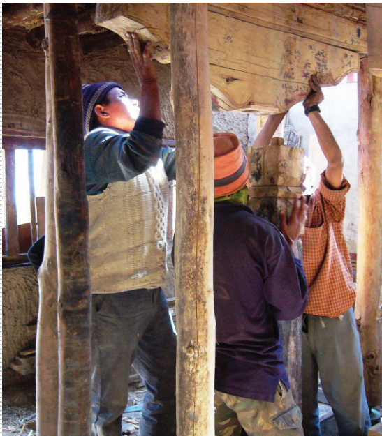
REALIGNING THE CENTRE PILLAR IN THE CHAPEL AFTER JACKING UP THE MAIN BEAM UNDER THE ROOF LANTERN
