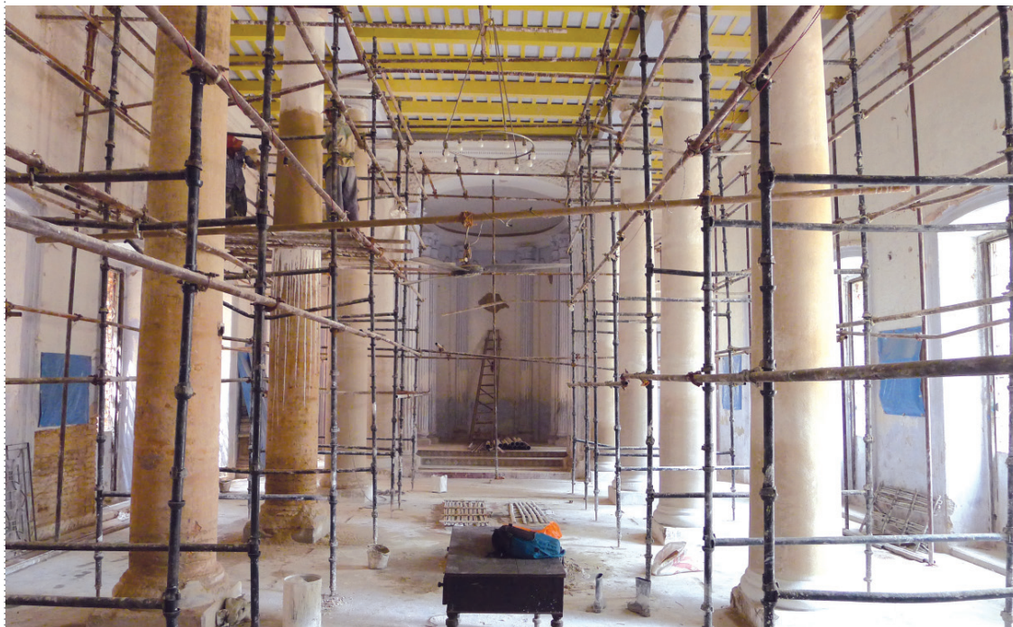
PAINT WORK IN PROCESS ON THE INTERIOR COLUMNS
