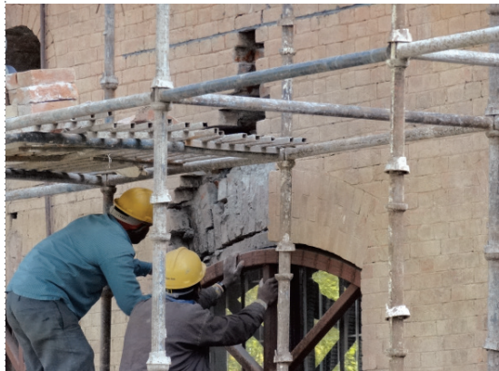
REPAIRING MASONRY ARCH
