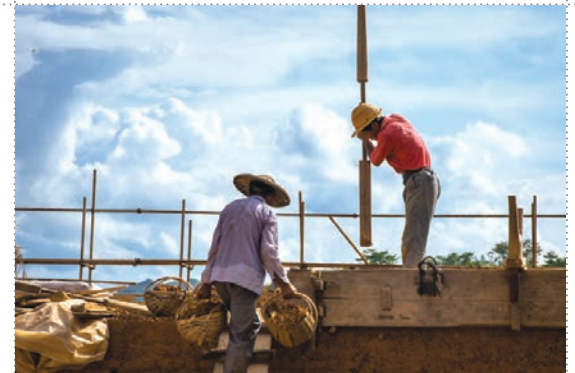
WORK IN PROGRESS ON THE RAMMED-EARTH WALL
