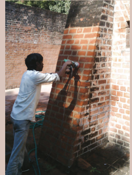
SPECIALIZED CLEANING OF THE BRICK FAÇADE
