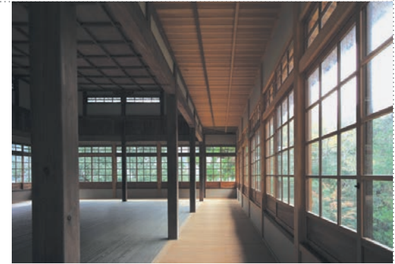
THE INTERIOR OF THE HALL BEFORE AND AFTER RESTORATION. MOST OF THE ORIGINAL GLASS WAS RETAINED AND REUSED.
