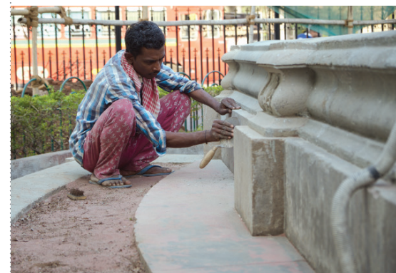
REMOVING PAINT FROM THE GROUND TROUGH
