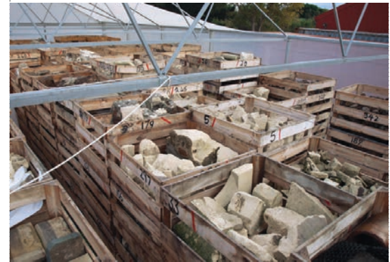
ORIGINAL STONWORK WAS RETRIEVED AND ABLE TO BE INCORPORATED INTO THE RECONSTRUCTION
