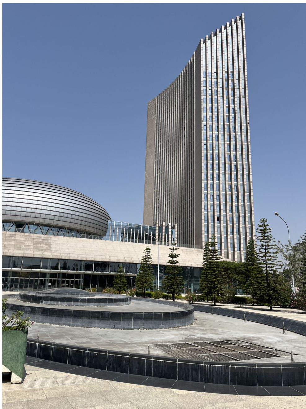
Figure 1. Tongji University Architectural Design Institute (Ren Lizhi), African Union Conference Center and Office Complex, Addis Ababa, 2012. Photograph by Kenny Cupers.
