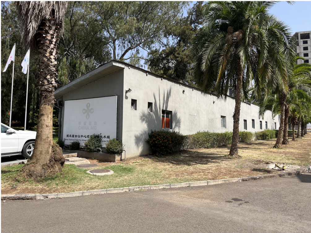
Figure 14. Office of the Chinese facilities management team on the site of the African Union Conference Center and Office Complex, 2022. Photograph by Kenny Cupers, 2022.
