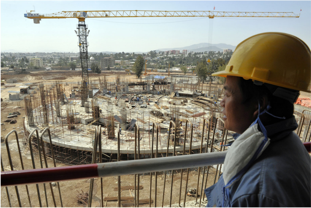
Figure 12. African Union Conference Centre and Office Complex under construction, 2010. Getty Images.
