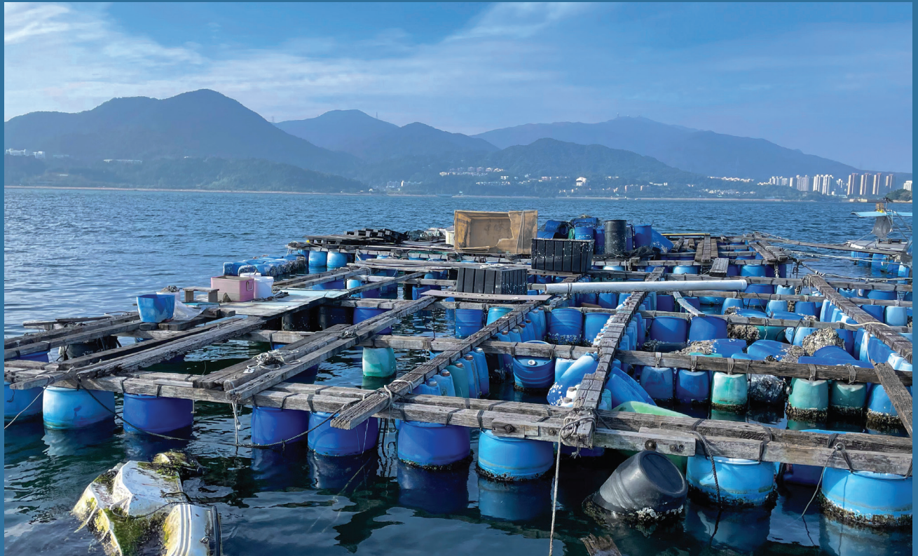
Figure 44 The group revitalized old and idle mariculture raft to be powered by solar energy.
