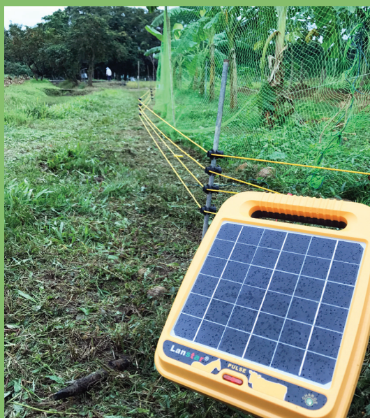
Figure 9 Solar powered electric fence at Lai Chi Wo.
