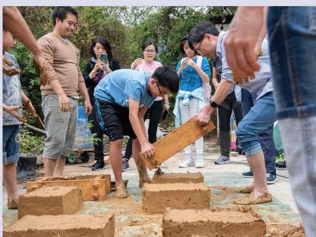
Figure 72 The group also offered workshops on adobe brick making. (Photo by Art for All- Murmur of the Brick – Rurally Engaged Art)
