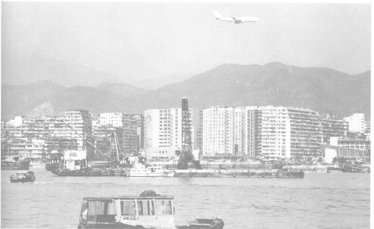
Plate 3 Proximity of the works to sensitive receivers in the Kowloon hinterland.
