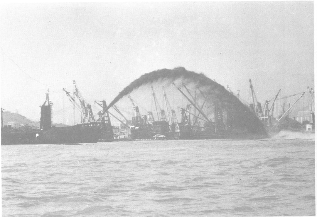
Plate 1 Rainbowing sand from a large dredger to form the reclamation.
