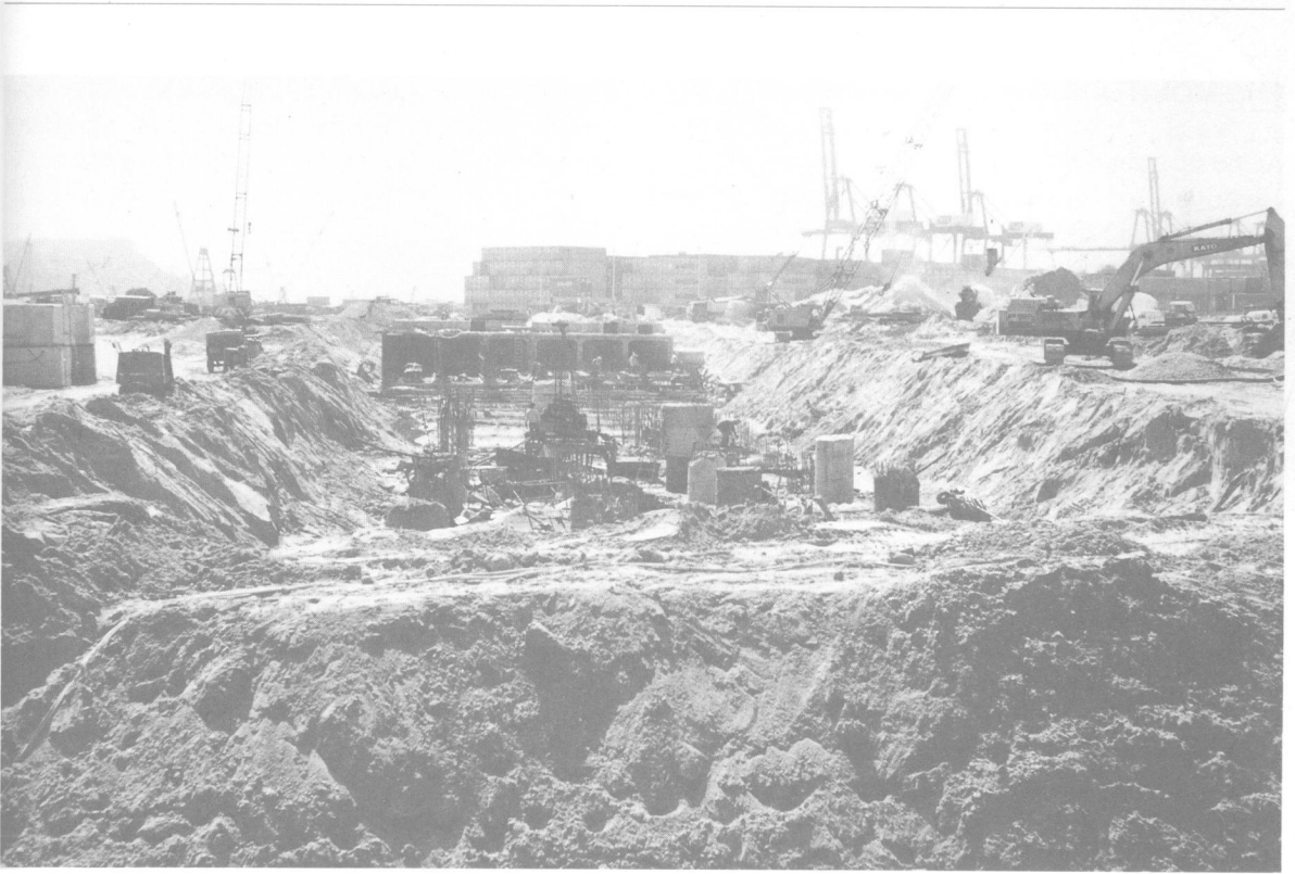
Plate 2 Formation of a multiple-cell box culvert on the West Kowloon Reclamation.
