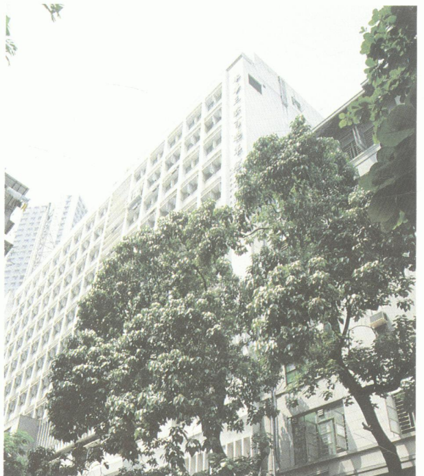
The Centenary Block of Tung Wah Hospital
