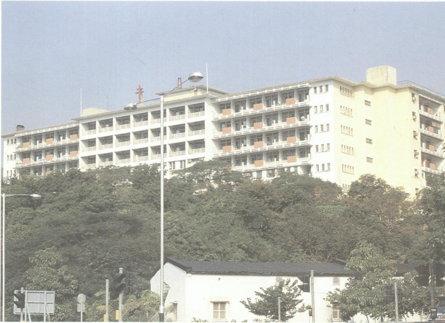
The original building of The Grantham Hospital
