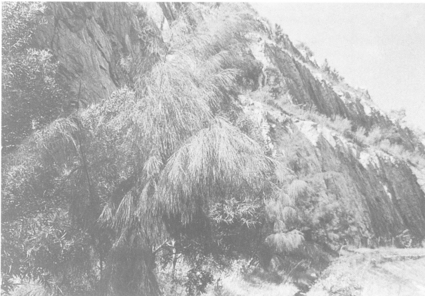
Fig. 9. View of the formed bench slope at Lam Tei Quarry
