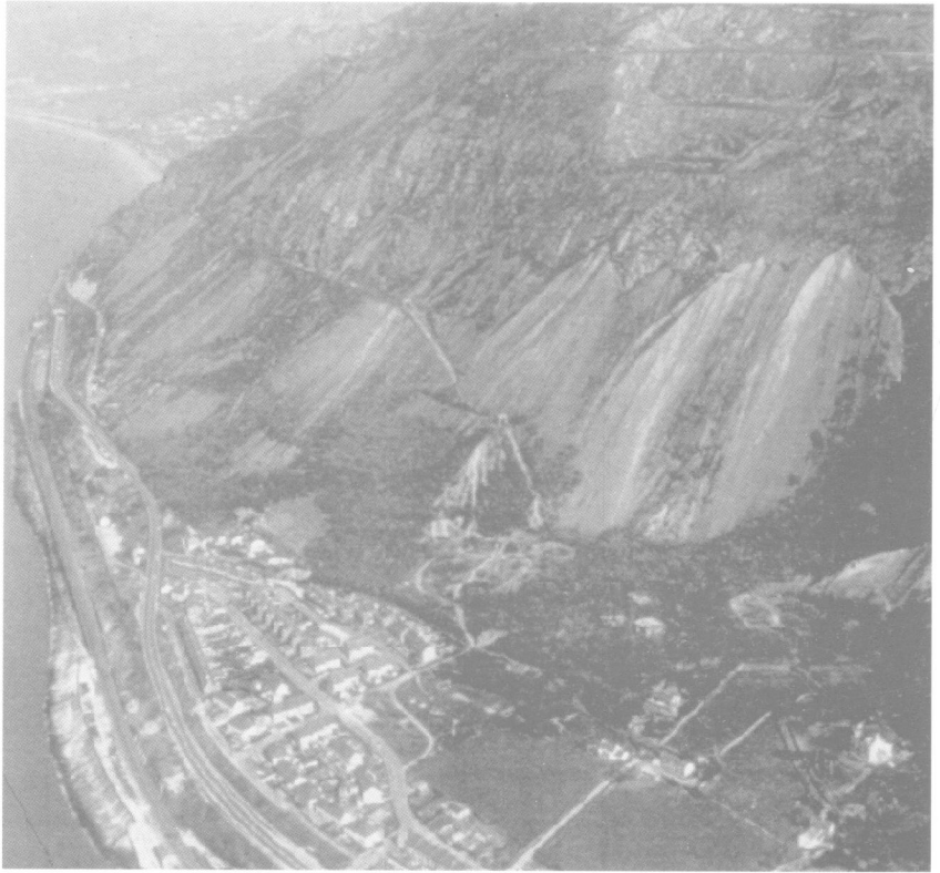
Fig. 10. The Pen-Y-Clip headland tunnel collapse. Soil-infilled vertical fractures led to the soil collapsing into the tunnel and a chimney extending up to the surface of the hillside above
