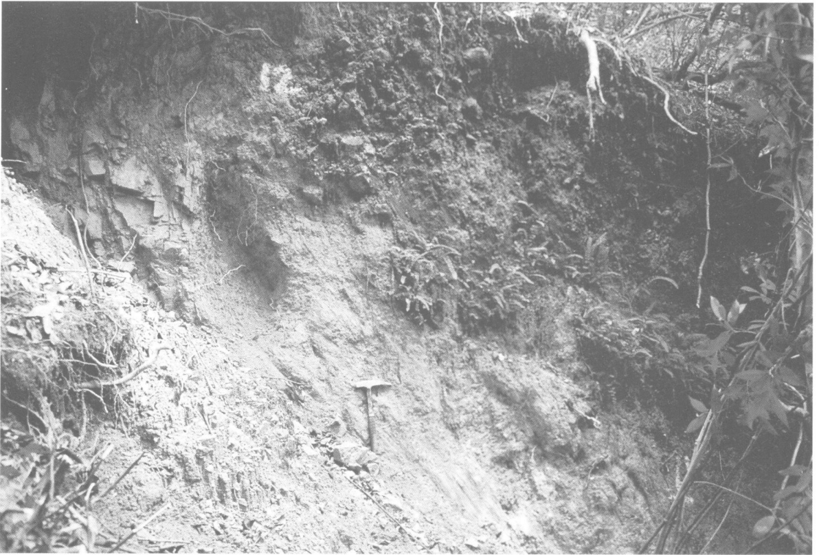
Fig. 6. Main scarp showing vegetation line indicating at least two phases of movement together with old and recent slickensides on the scarp surface and a rhyolite dyke contact (taken 26 September 1997)
