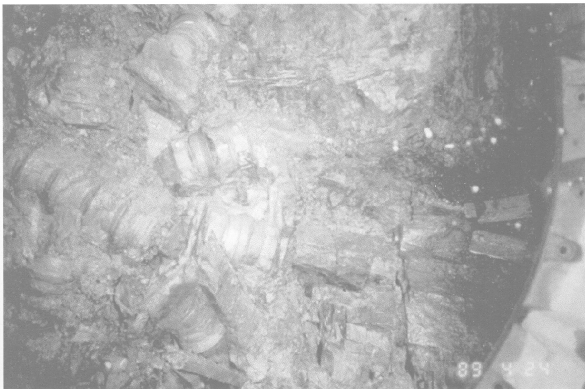
Fig. 13 (below). Tunnel collapse after encountering a fault zone. The extent and weaknesses of the fault zone had not been anticipated even though it was known from ground investigation that a fault occurred at that location.
