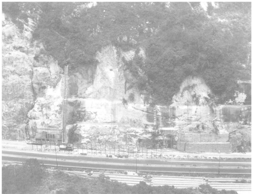
Fig. 15. Landslide on Tuen Mun Highway, Hong Kong where failure was interpreted as having been caused by perching of water above a gently dipping dolerite dyke
