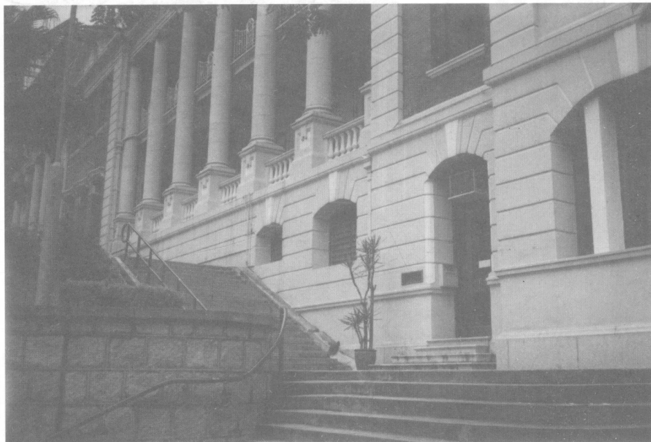
The Main Campus Room 1, University Office at the Main Building Corner
