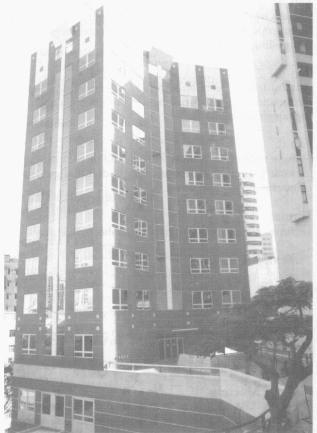
In May '96 SPACE moved into brand new headquarters
